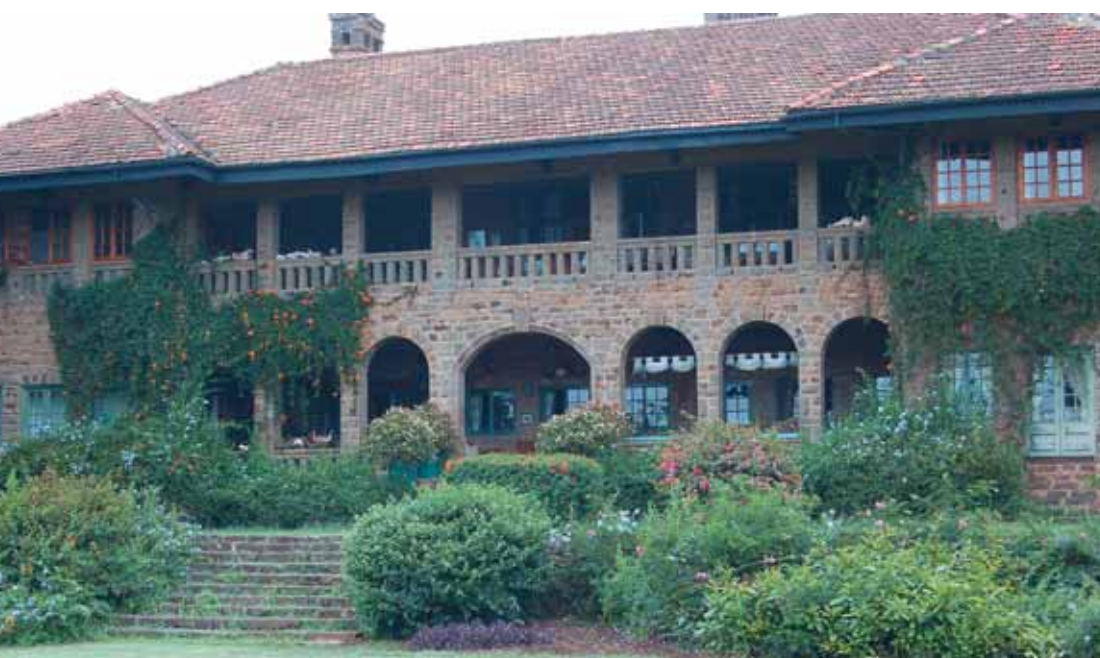
Deloraine, Voorspuy's home built by Lord Francis Scott
