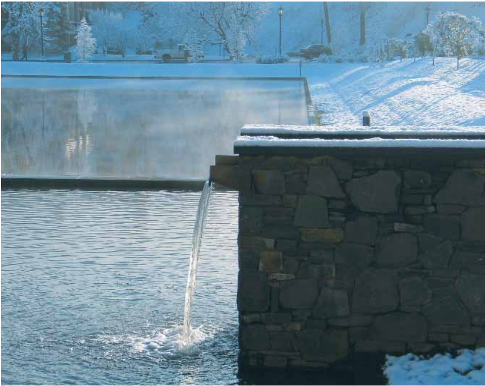
Water enters the forebay via a spillway, creating varying arcs of water that change with rainfall and the seasons.
