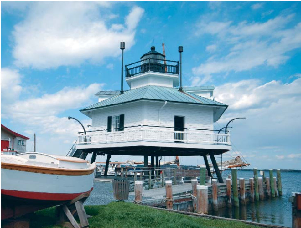
The Chesapeake Maritime Museum in St. Michaels is home to the former Hooper Strait Lighthouse. The once-condemned lighthouse was barged 60 miles to its current location in 1966.
